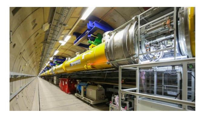
A view into the main accelerator tunnel of European XFEL, where 100 superconducting accelerator modules are being installed. Credit: Dirk Nölle, DESY
