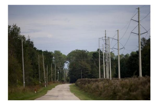
In this Nov. 12, 2015 photo, concrete poles carrying feeder lines, right, line the roadway with traditional wooden electrical poles at left, near the Stennis substation for Coast Electric, which has been built up to a higher elevation, in Kiln, Miss. Utilities across the country are struggling to balance customer costs with the need for improvements to counter the rising number of violent storms, floods and droughts threatening the U.S. power grid's core infrastructure. (AP Photo/Gerald Herbert)
