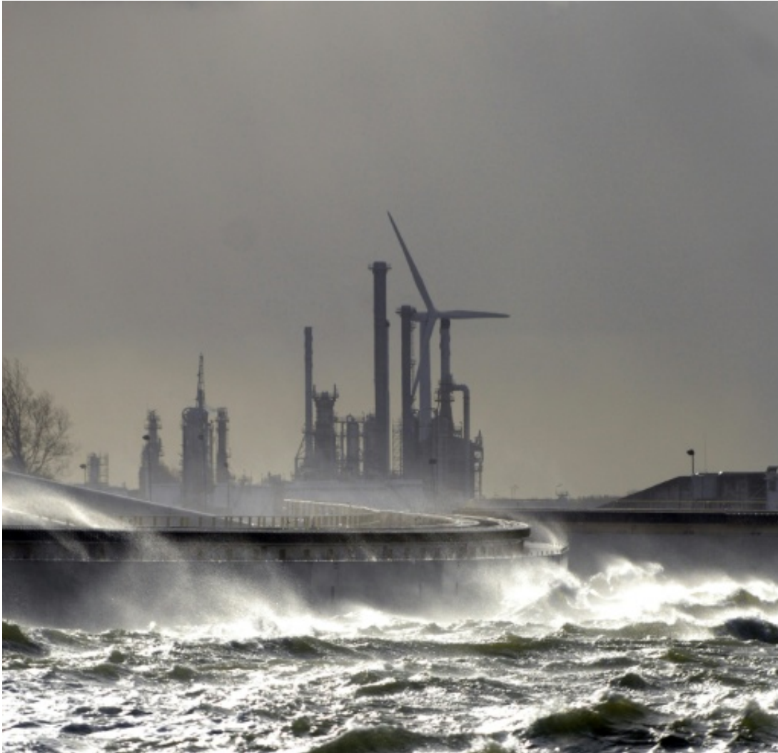
The giant Maeslant surge barrier that guards the entrance to the largest port in Europe, Rotterdam
