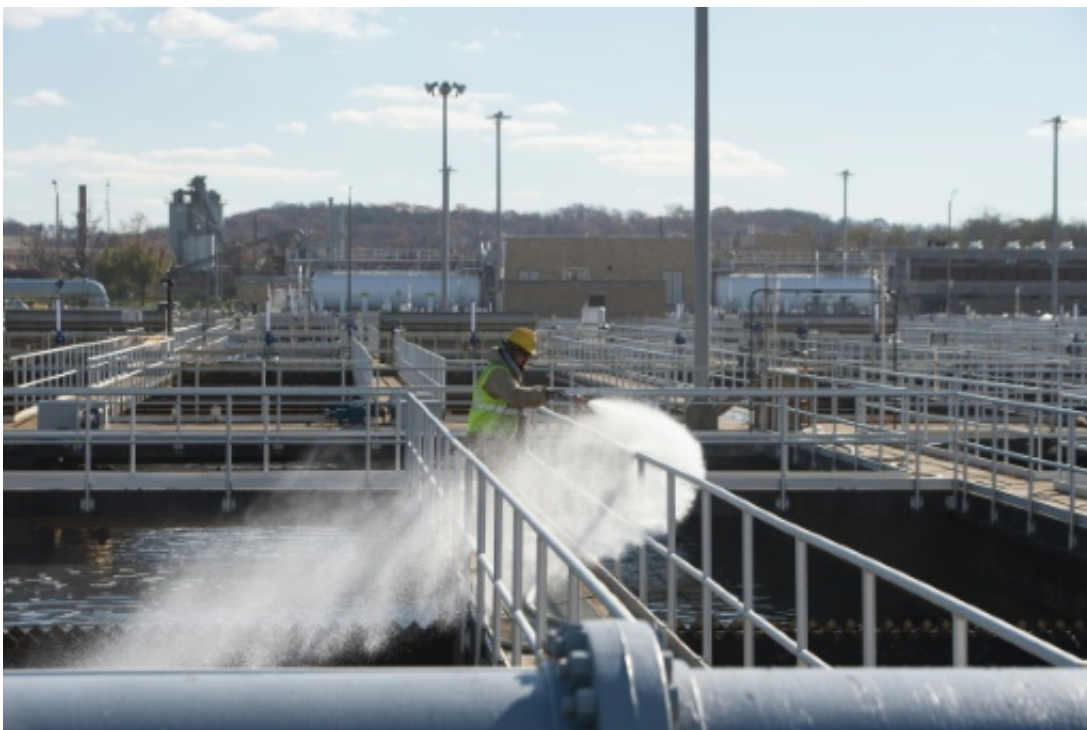
A worker is seen cleaning a wastewater pool at DC Water's Blue Plains plant in Washington, DC
