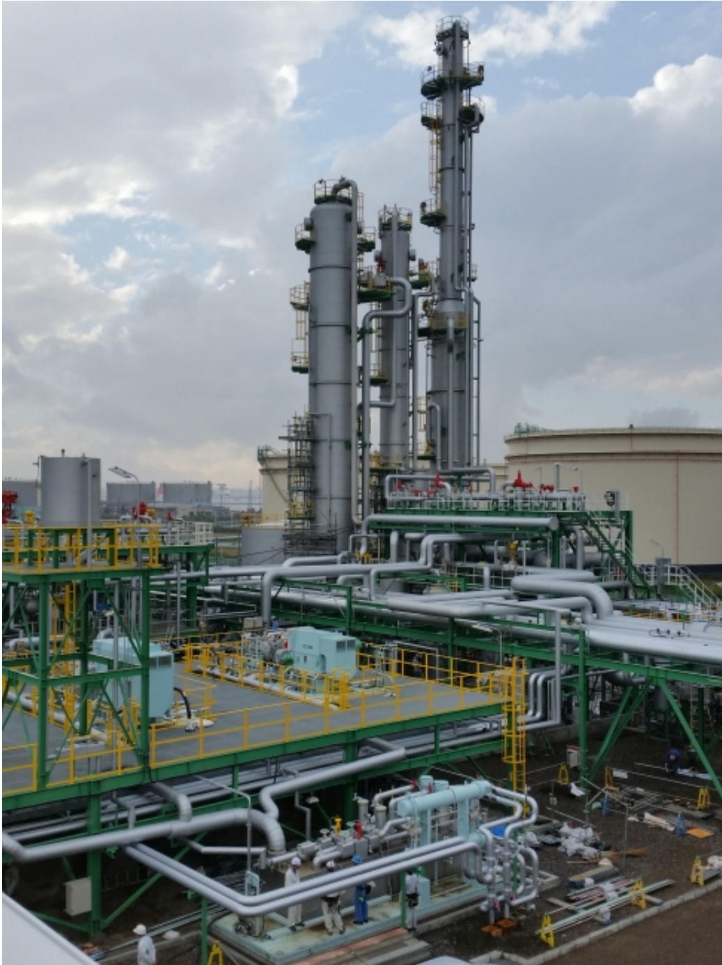
The Carbon Capture and Storage (CCS) demonstration facility in Tomakomai, Hokkaido, Japan. This view shows the carbon dioxide absorption and separation towers. Credit: Florian Kraxner
