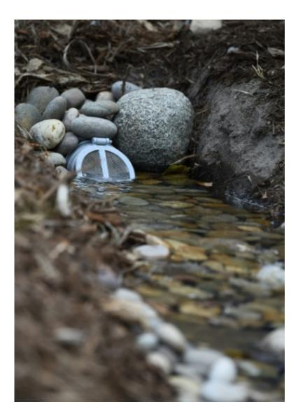
A newly installed "rain garden," part of drought-alleviation measures in Los Angeles, helps storm overflow captured from a residential rooftop filter gradually into the ground and water table rather than allowing it to go down storm sewers to the sea
