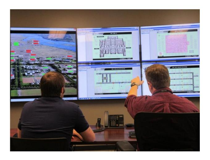
The Building Operations Control Center at PNNL will act as the nerve center monitoring and controlling information on energy usage at multiple campuses in Washington state to research and test transaction based energy usage in and between buildings. Credit: PNNL
