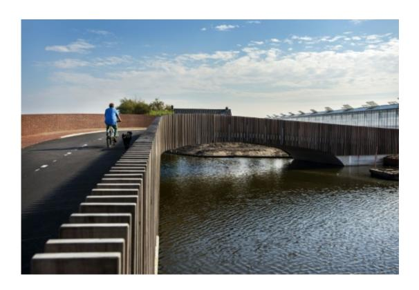
The "batbridge" in the Dutch town of Monster is designed with special cavities for bats to hunker down in to hibernate or reproduce
