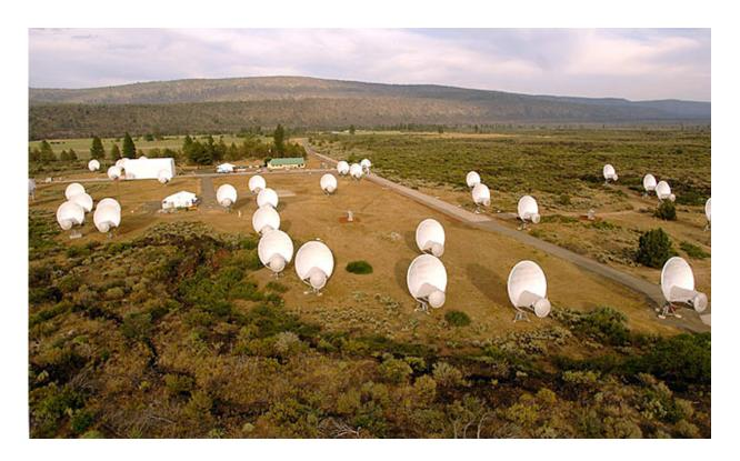
The Allen Telescope Array (ATA) is a "Large Number of Small Dishes" (LNSD) array designed to be highly effective for simultaneous surveys undertaken for SETI projects (Search for Extraterrestrial Intelligence) at centimeter wavelengths. Credit: Seth Shostak / SETI Institute
