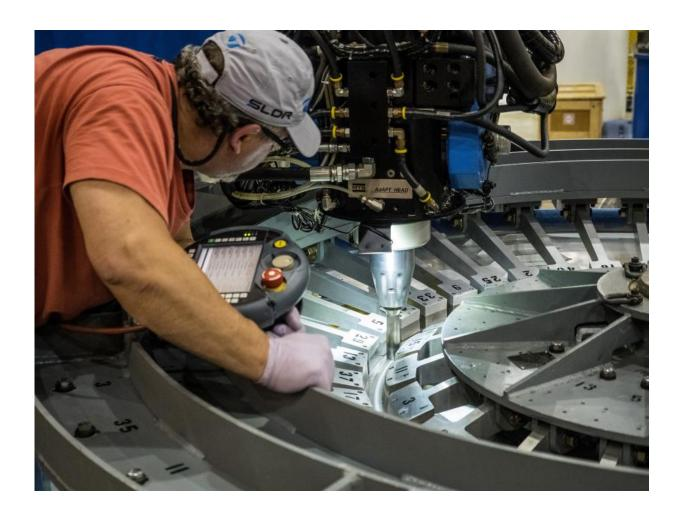
At NASA's Michoud Assembly Facility in New Orleans, engineers welded together on Sept. 5, two sections of the Orion spacecraft's primary structure that will fly on Exploration Mission-1, the first flight of Orion atop the agency's Space Launch System rocket. Credit: NASA
