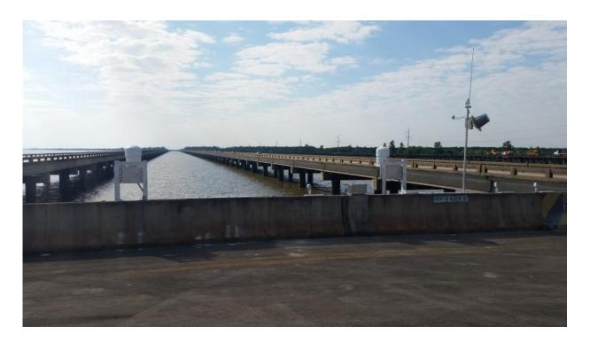
The new NOAA water and meteorological station on the western side of Lake Pontchartrain is built to withstand winds of up to 110 miles per hour. Credit: NOAA
