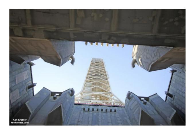
Looking up from beneath the enlarged exhaust hole of the Mobile Launcher to the 380 foot-tall tower astronauts will ascend as their gateway for missions to the Moon, Asteroids and Mars. The ML will support NASA's Space Launch System (SLS) and Orion spacecraft during Exploration Mission-1 at NASA's Kennedy Space Center in Florida. Credit: Ken Kremer/kenkremer.com
