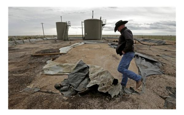
In this April 24, 2015 photo, Justin Johnson looks at a torn lining at a tank and pipeline station adjacent to his ranch near Crossroads, N.M. Trucks bring oilfield wastewater to the station, where it is pumped through pipelines to a disposal well. The lining is intended to prevent wastewater from seeping into the ground in the event of a leak, but it is in poor condition. (AP Photo/Charlie Riedel)
