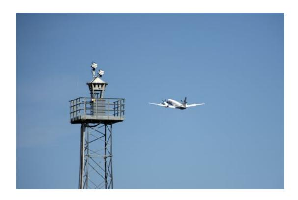
In this April 2015 photo provided by Saab AB, a plane takes off beyond a remotely controlled control tower at Ornskoldsvik Airport in northern Sweden. The dozen commercial planes that land here each day are guided in by controllers using video cameras at another airport 90 miles away. It's the first airport in the world to use such technology, but others in Europe are testing the idea as is one airport in the United States. (Stefan Kalm/Saab AB via AP)
