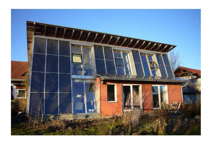
Solar-Active-Houses get most of their heat from the sun. Researchers carried out scientific tests to explore how this energy concept can be optimized further. Credit: Fraunhofer ISE
