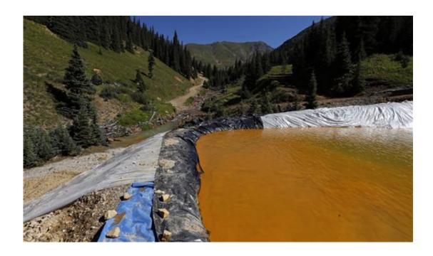
Water flows through a series of sediment retention ponds built to reduce heavy
