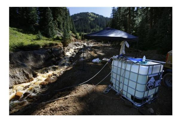
A plastic container feeds additives through tubes into mine wastewater flowing into a series of sediment retention ponds, part of danger mitigation in the
