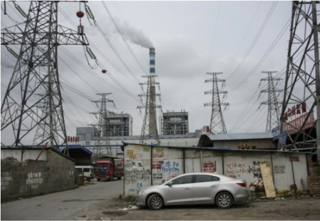
Smoke rises from a tower in Shanghai Wujing Chemical Industrial Park on July 17, 2015
