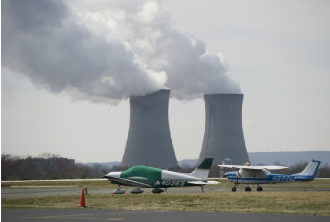
Cooling towers at the Limerick nuclear power plant in Pottstown, Pennsylvania
