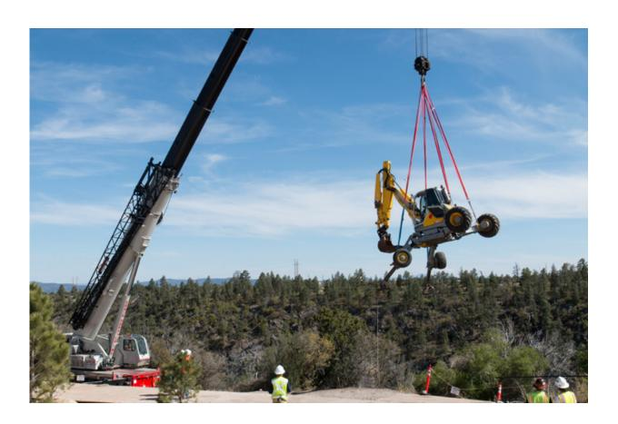
A telescoping crane hoists a spider excavator over Los Alamos Canyon before placing it on the canyon slope to excavate historically contaminated soil.
