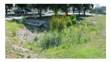
The bioretention/rain garden area the the Texas A&M AgriLife Research and Extension Center in Dallas handles stormwater runoff from a 37,000-square-foot parking lot at the facility. Credit: Texas A&M AgriLife Extension Service photo
