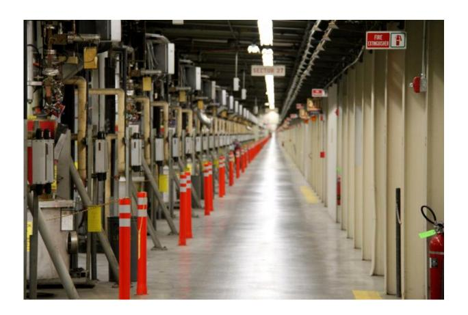
SLAC's Klystron Gallery is a nearly 2-mile-long building that sits above the linear accelerator. The Klystron Gallery houses hundreds of klystrons that generate microwave pulses used as accelerating energy for the electron beam. Originally built for particle physics experiments, the linac now supplies electron beams that are used to generate ultrabright X-ray pulses for SLAC's Linac Coherent Light Source. Credit: SLAC National Accelerator Laboratory
