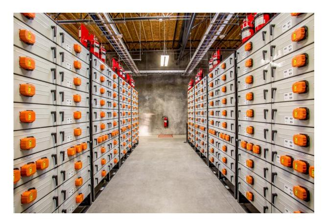
Portland General Electric installed a 5-megawatt, lithium-ion battery in Salem, Oregon, as part of the Pacific Northwest Smart Grid Demonstration Project. Credit: Portland General Electric
