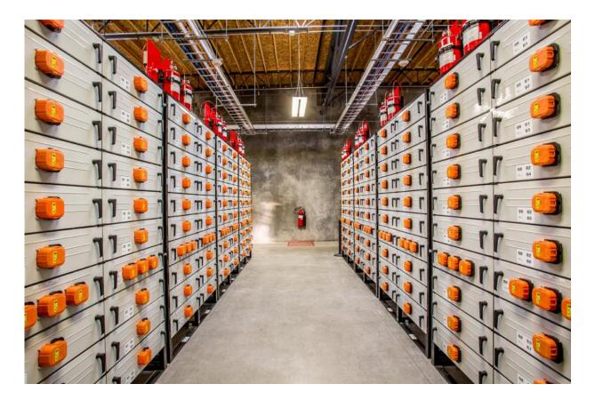
Portland General Electric installed a 5-megawatt, lithium-ion battery in Salem, Oregon, as part of the Pacific Northwest Smart Grid Demonstration Project. Credit: Portland General Electric
