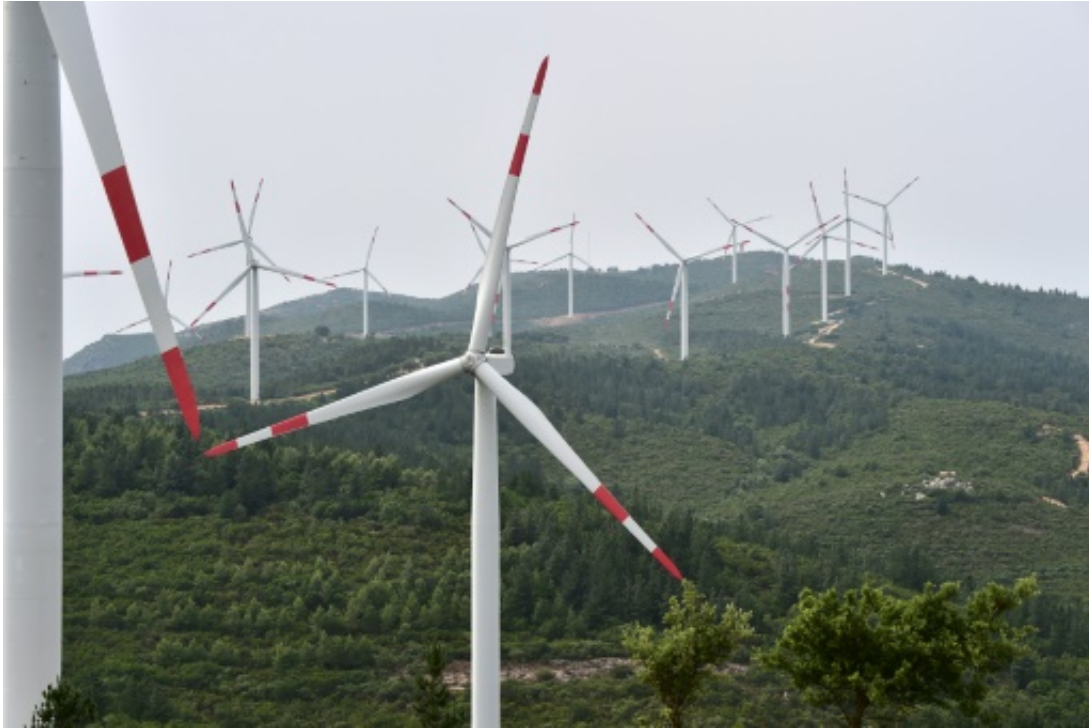
Wind turbines in a wind farm near Oristano in Sardinia
