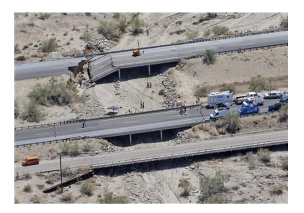
This aerial photo shows the collapsed elevated section of Interstate 10, Monday, July 20, 2015, in Desert Center, Calif. All traffic along one of the major highways connecting California and Arizona was blocked indefinitely when the bridge over a desert wash collapsed during a major storm, and the roadway in the opposite direction sustained severe damage. (AP Photo/Matt York)
