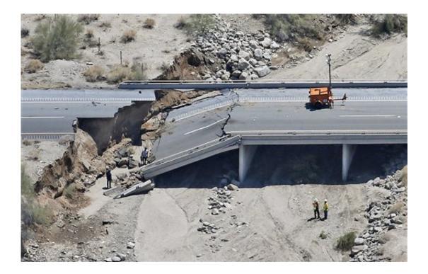
This aerial photo shows the collapsed elevated section of Interstate 10, Monday, July 20, 2015, in Desert Center, Calif. All traffic along one of the major highways connecting California and Arizona was blocked indefinitely when the bridge over a desert wash collapsed during a major storm, and the roadway in the opposite direction sustained severe damage. (AP Photo/Matt York)
