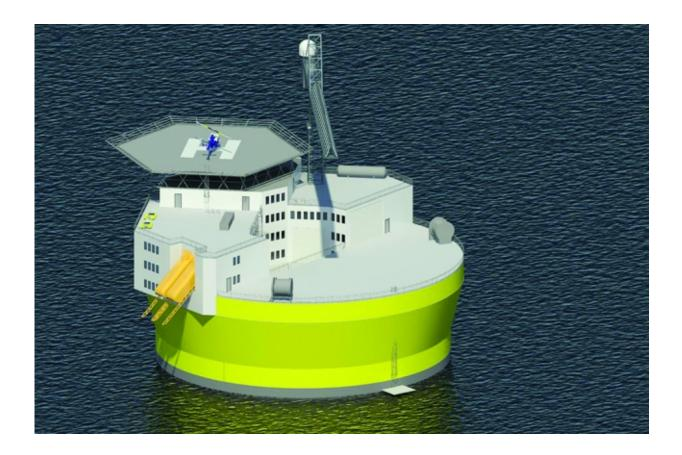
The proposed Offshore Floating Nuclear Plant structure is about 45 meters in diameter, and the plant will generate 300 megawatts of electricity. An alternative design for a 1,100 MW plant calls for a structure about 75 meters in diameter. In both cases, the structures include living quarters and helipads for transporting personnel, similar to offshore oil drilling platforms.
