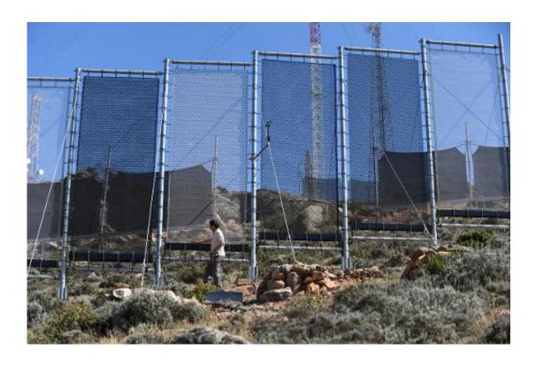
Thick fog is trapped by finely meshed panels and relayed it to a network of pipes
