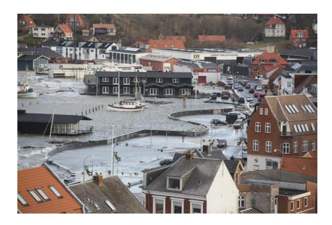
Lemvig in western Jutland, Denmark has coastal protection in the form of a curved concrete wall that winds across the harbour area. The high water wall functions optimally against high water levels up to 2.10 meters and it already proved its worth during a large storm in December 2013. When there is no storm warning, the wall's sliding doors open and create an attractive area at the harbor with a promenade, benches and gathering places. Credit: Mads Krabbe
