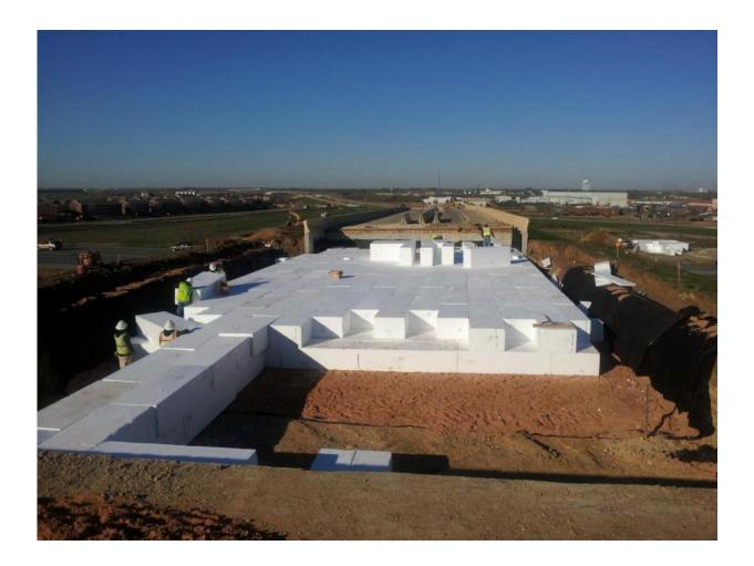
Geofoam blocks being installed underneath a North Texas highway will ensure stability for a longer period of time than traditional construction. Credit: UT Arlington
