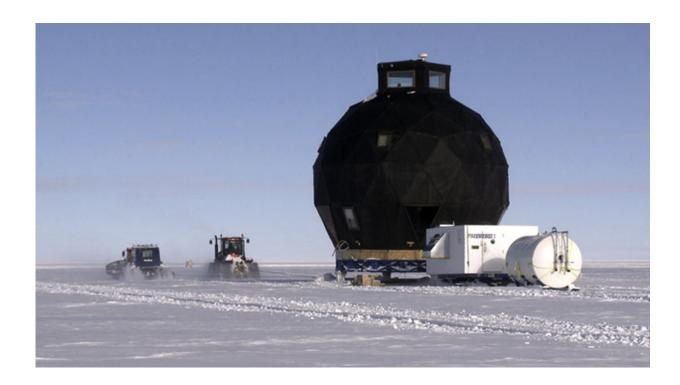
The 14-meter high building, the 'Dome', weighing 47 tons, is on skis and is being pulled across the snow by two tracked vehicles.
