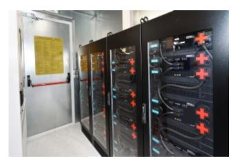
The batteries store solar power and feed it into the mains of HIU, if required. Credit: Frederik Elschenbroich
