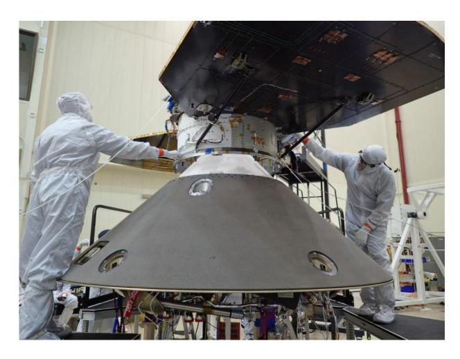
Spacecraft specialists at Lockheed Martin Space Systems, Denver, are preparing to attach the cruise stage of NASA's InSight spacecraft to the top of the spacecraft's back shell in this April 29, 2015, photo. The cruise stage will serve multiple functions during the flight from Earth to Mars. It has its own solar arrays, thrusters and radio antennas. It will be jettisoned shortly before the spacecraft enters the Martian atmosphere. Credit: NASA/JPL-Caltech/Lockheed Martin
