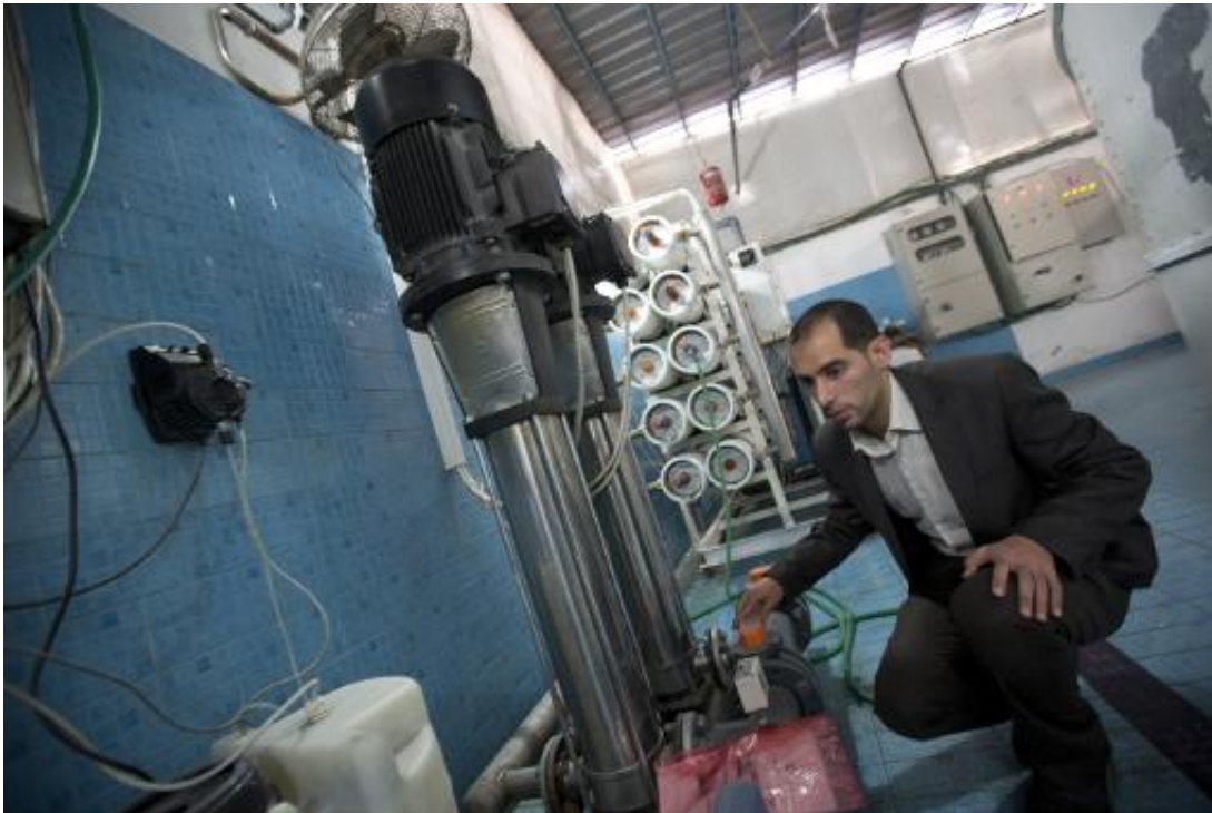
Palestinian engineer Diao Abu Assi operates a machine that makes seawater potable in Gaza city
