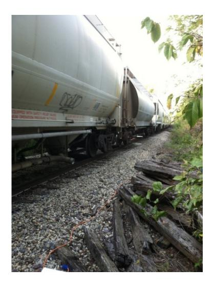
The big chunks of rock that keep railroad tracks in place look like a solid footing, but temperature and vibration can destabilize ballast over time. Credit: Tuncer Edil/UW-Madison
