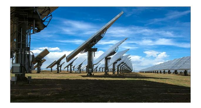
Utility-scale solar power is growing quickly in the United States—but increasingly, investors want assurance of the reliability of the panels, modules, and complete systems before they invest tens of millions of dollars in the projects. Shown here is the Alamosa Solar Generating Project, the first large (30-megawatt) high concentration solar PV power generation system in the world, located on 225 acres in the San Luis Valley near Alamosa, Colorado. Credit: Dennis Schroeder
