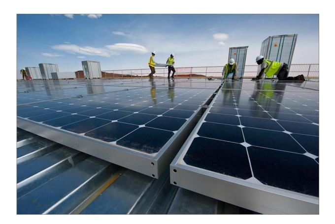
Work by Namaste Solar installing PV modules on the roof of the parking structure on NREL's South Table Mountain campus. The finished product includes 3,632 solar modules installed on the garage roof and south facade. Credit: Dennis Schroeder
