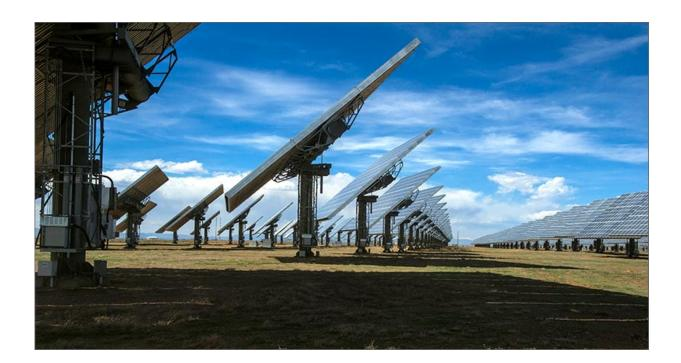
Utility-scale solar power is growing quickly in the United States—but increasingly, investors want assurance of the reliability of the panels, modules, and complete systems before they invest tens of millions of dollars in the projects. Shown here is the Alamosa Solar Generating Project, the first large (30-megawatt) high concentration solar PV power generation system in the world, located on 225 acres in the San Luis Valley near Alamosa, Colorado. Credit: Dennis Schroeder
