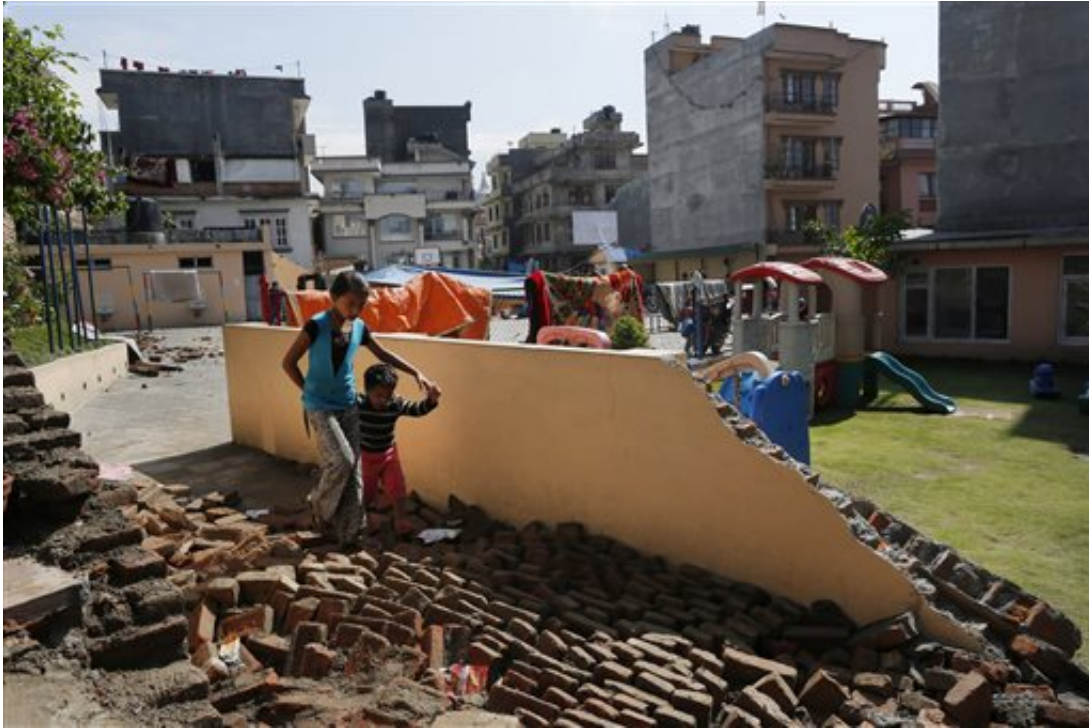
A young girl walks with a boy over a collapsed school playground in Kathmandu, Nepal, Monday, April 27, 2015. A strong magnitude 7.8 earthquake shook Nepal's capital and the densely populated Kathmandu Valley on Saturday, causing extensive damage with toppled walls and collapsed buildings. (AP Photo/Wally Santana)
