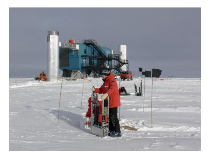
Jason Koskinen at the South Pole. In the background is the IceCube Lab. All data from the instruments deep down in the ice comes up through the two 'towers' and into the computer center, where the first analyses are done. Credit: T. Waldemaier
