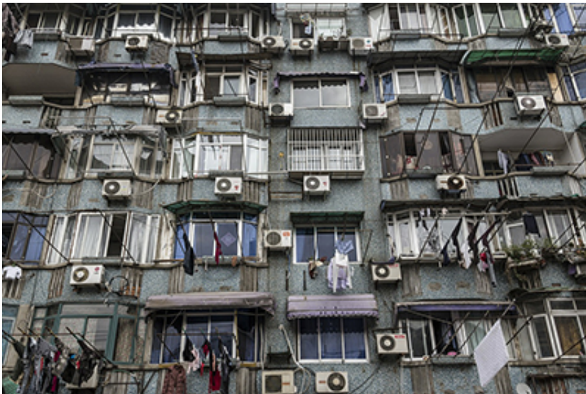
Air conditioners in China. Credit: Berkeley-Haas
