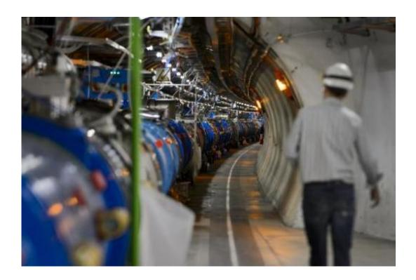
The Large Hadron Collider comprises a ring-shaped tunnel straddling the Franco-Swiss border, in which two beams of protons are sent in opposite directions
