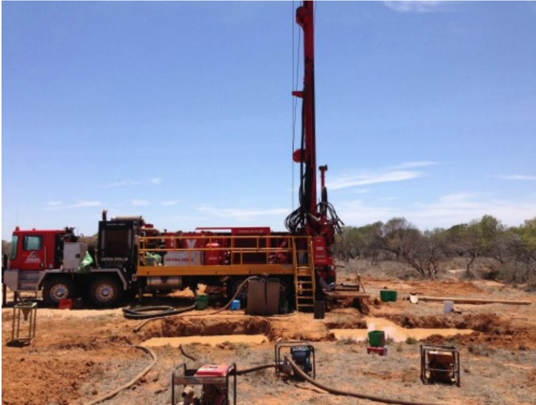
Installing water production bores at Carnarvon. Credit: DAFWA
