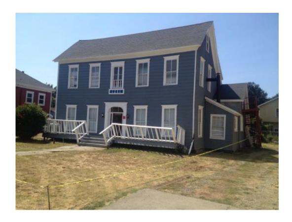
Damage from M 6.0 earthquake to older building in City of Napa. Credit: Erol Kalkan, USGS and guest editor of SRL special issue on South Napa quake.
