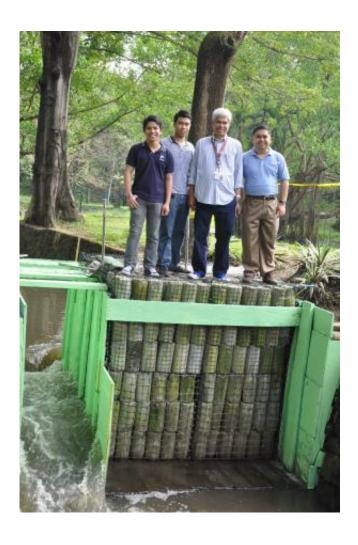
The dam's frame consists of gabion cages: wire mesh baskets filled with sturdy columns of recycled concrete cylinders or rocks.
