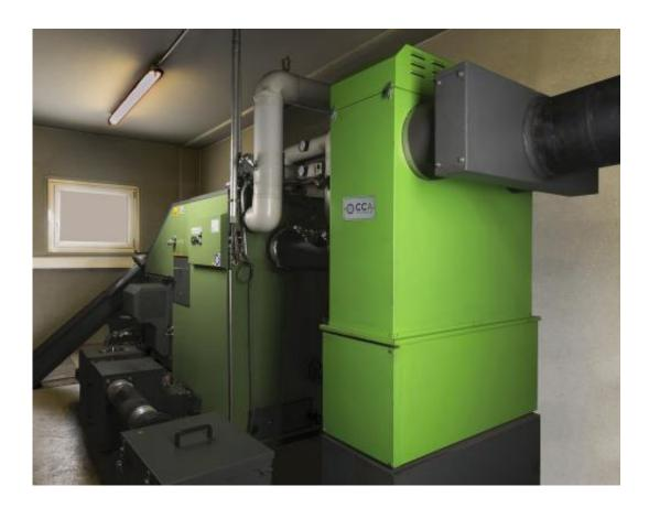
The Carola-precipitator (light green) is installed into the flue gas passage reduces the concentration of soot and fine dust by up to 90%. Credit: KIT/P. Langer
