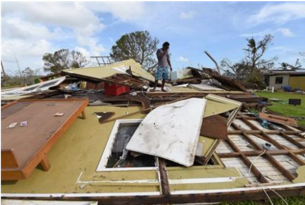
Adrian Banga surveys his destroyed house in Port Vila, Vanuatu in the aftermath
