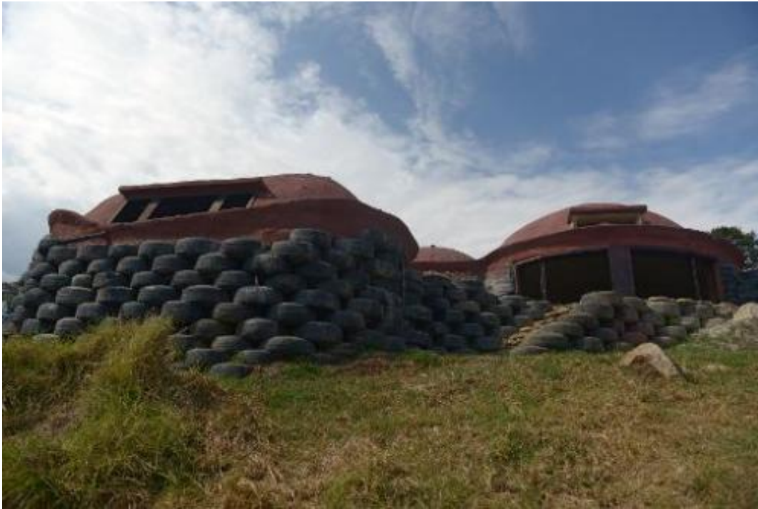
A view of a house built with discarded tires in Choachi, Cundinamarca, Colombia on March 16, 2015
