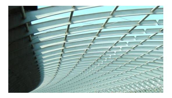
The Sound Tube in Melbourne, Australia is designed to reduce road noise. Credit: Wikimedia, CC BY-SA
