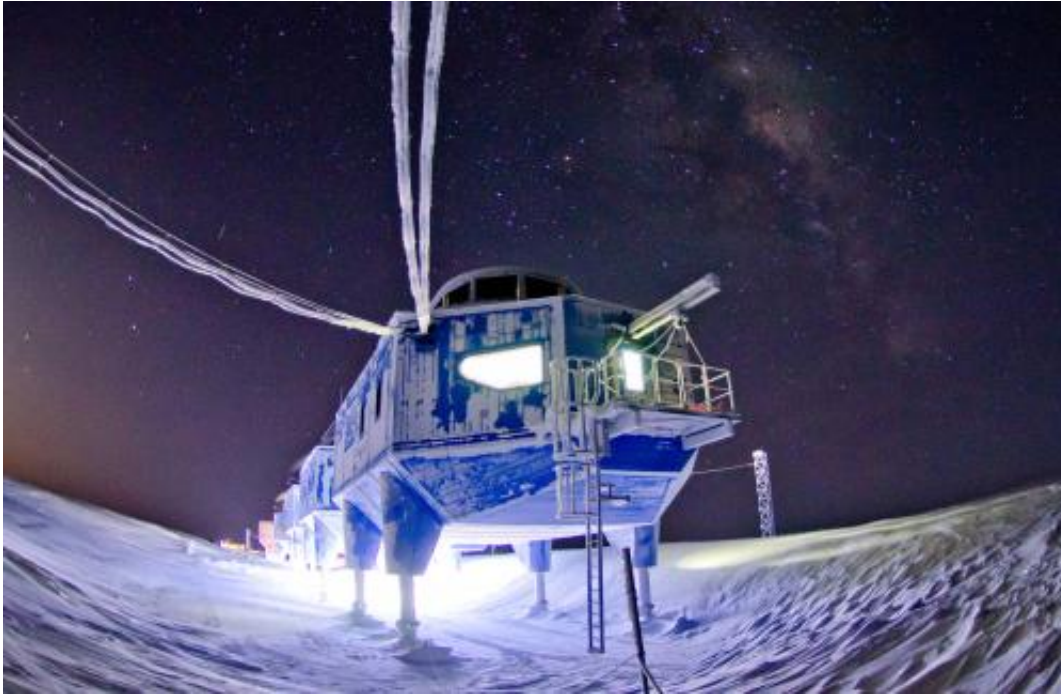
The British Antarctic Survey station Halley VI.
