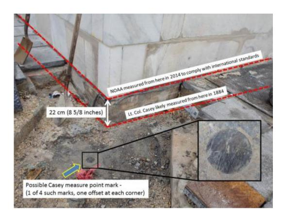
Illustration of the measuring points used by Lt. Col. Thomas Casey in 1884 and the 2014 measuring point used by NOAA to meet CTBUH standards. Credit: NOAA
