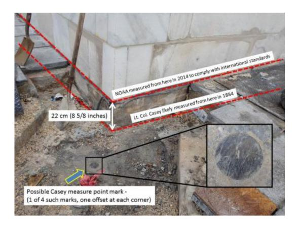
Illustration of the measuring points used by Lt. Col. Thomas Casey in 1884 and the 2014 measuring point used by NOAA to meet CTBUH standards. Credit: NOAA
