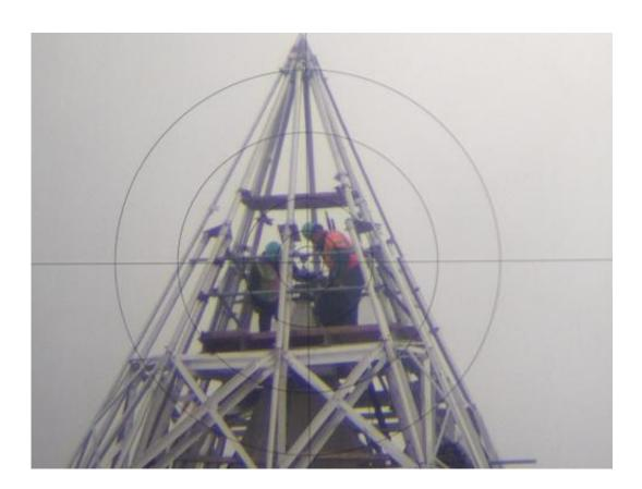
The view of the top of the Monument as viewed through the Total Station surveying tool, captured by placing a smartphone camera up to the eyepiece.
