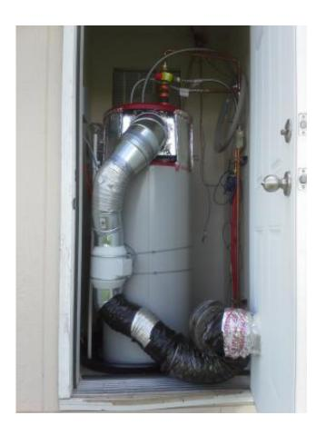
A fully ducted water heater, with ducting that collects air to warm water and exhausts used air outside. PNNL researchers found fully ducting a heat pump water heater reduced a home's total annual energy use by 4.2 percent, providing a \$1,982 10-year cost savings for a 1,500-square-foot home.
