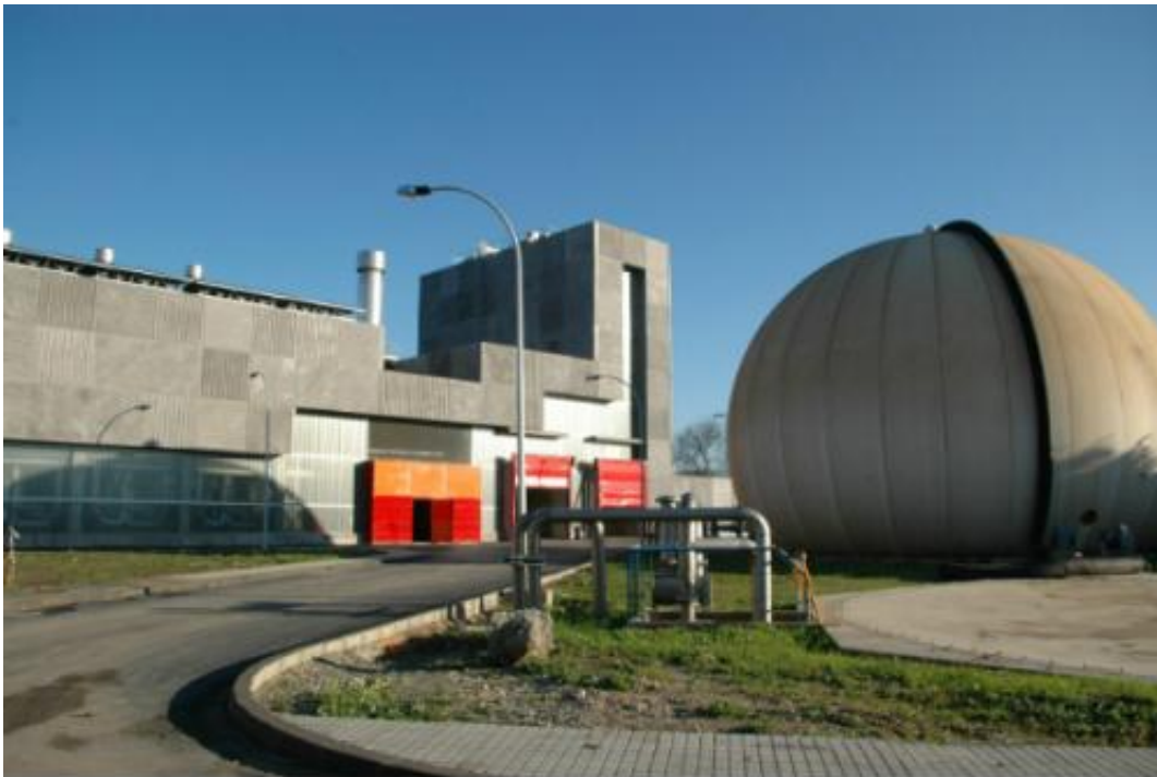
Thermal drying plant of sewage sludge at Guadalhorce/EMASA.
